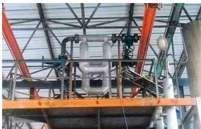
Figure 7-Actual installation of Coriolis meter
