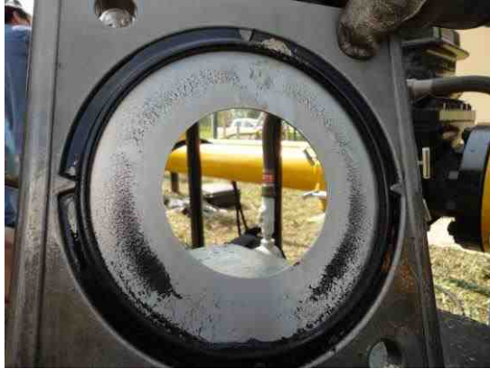
Figure 11 – Plate inspected during audit #2
