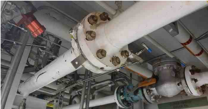
Figure 14 – Polar Lights 4” paddle plate orifice meter with diagnostics installed
