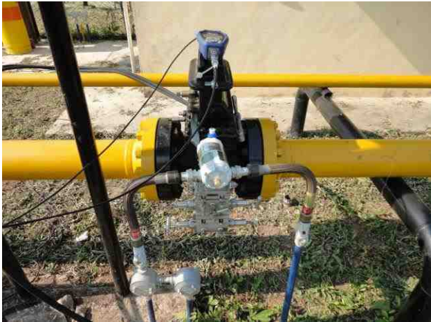
Figure 9 - 6" Orifice Meter run prior to audit #2
