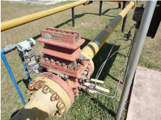
Figure 6 – 6" Orifice Meter run prior to audit #1
