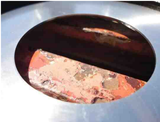
Figure 8 – Plate inspected during audit #1
