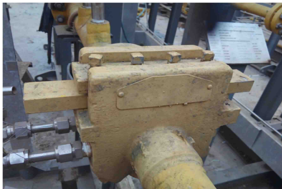
Figure2: Single chamber orifice fitting
